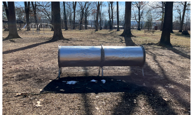
There is a lack of safety surfacing around this element. There are also sharp metal fittings & exposed bolts that could cause injury.
