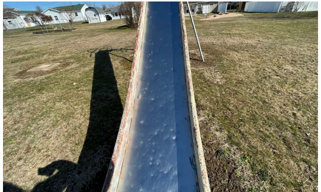
The metal slide surface with no shade can cause burns. There is also a lack of safety surfacing.
