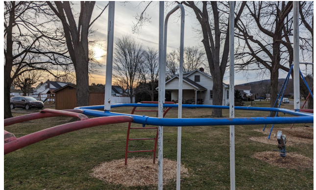
Exposed bolts protruding too far could cause injury. There is a lack of safety surfacing in the fall zone.
