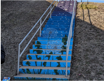
1 Stairs Mural, Jermaine Johnson Canal St
